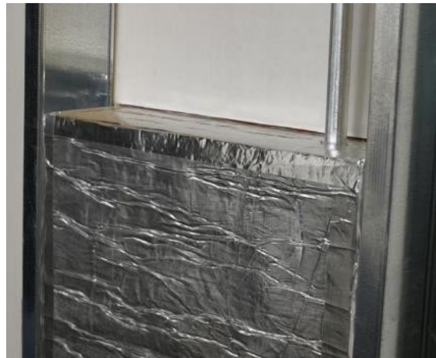
Box installed into wall cavity showing conduit
