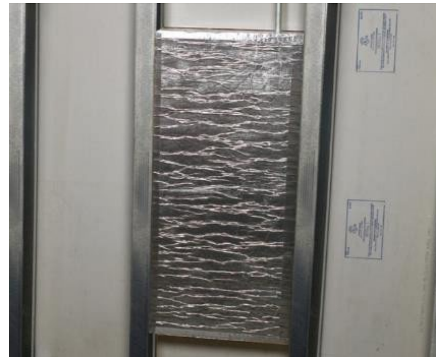
Box installed into wall cavity showing conduit
