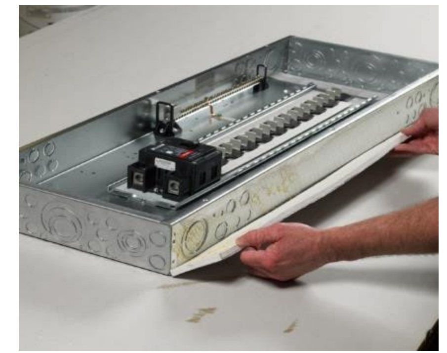
Applying mat to box sides
