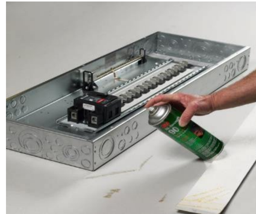
Applying adhesive to the box
