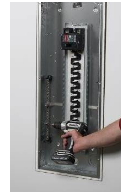
Securing box to the studs
