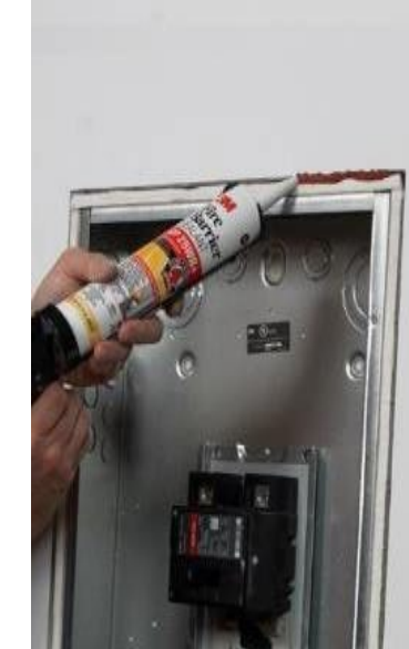
Applying sealant to mat and gypsum interface
