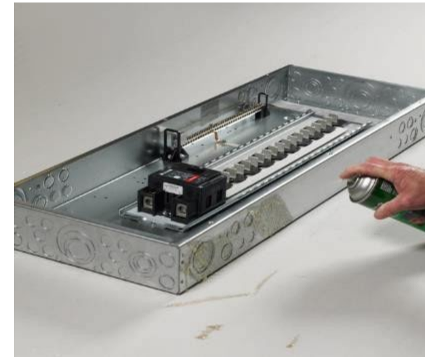
Applying adhesive to the box
