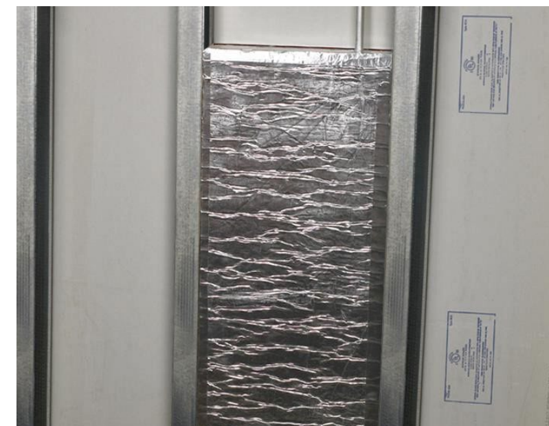
Electrical Panel Box
