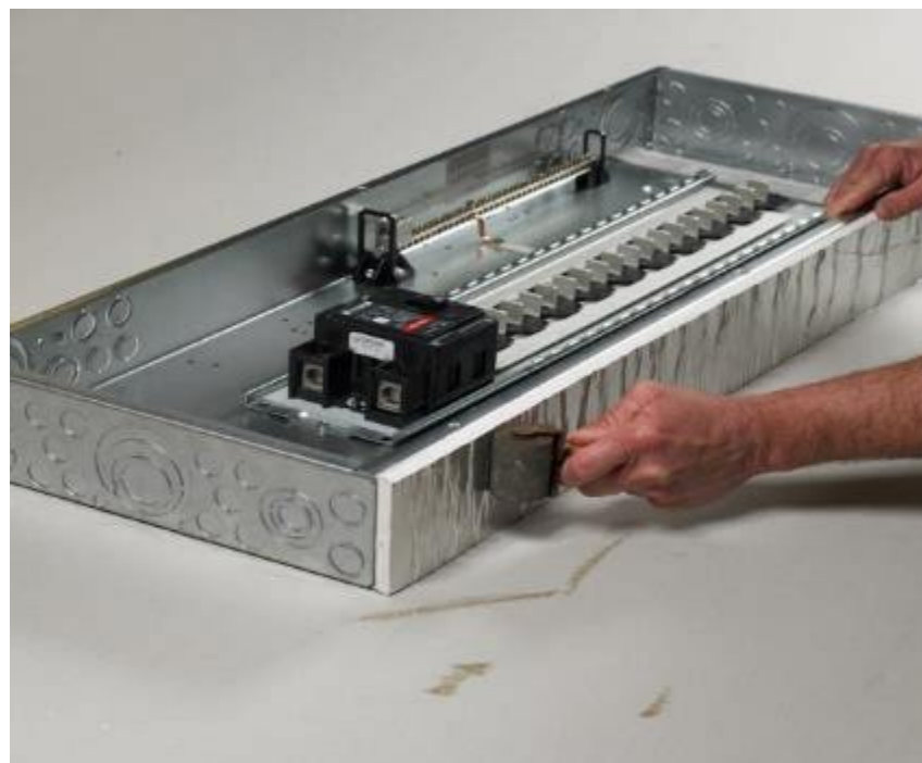
Securing mat to sides of box with roller
