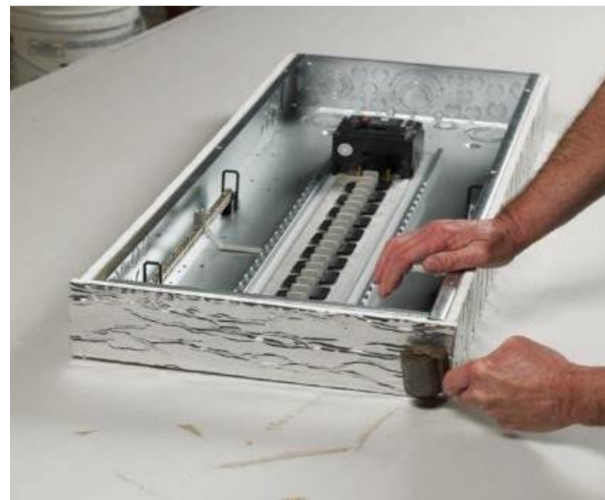
Securing mat to sides of box with roller
