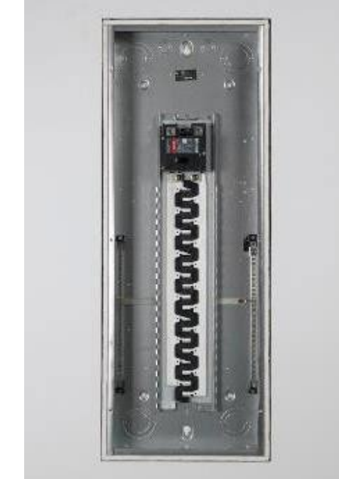
Box installed to studs
